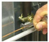
Unscrew the hollow screw connecting the thermocouple to gas valve using a wrench 8.
