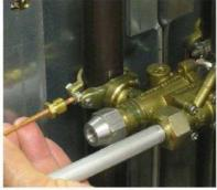
Remove the cell contact of the thermocouple to the gas valve.
